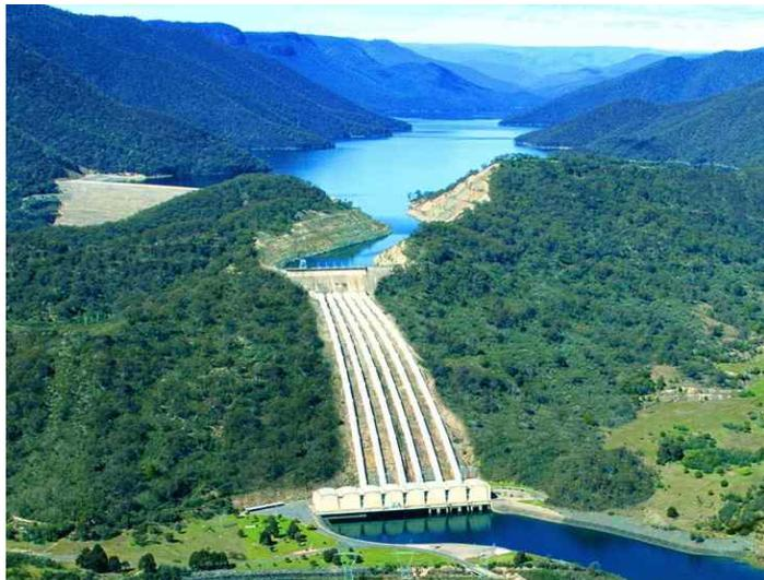
*Pumped hydro storage involves using excess energy to pump water uphill and then generating energy in the usual way when needed.*
